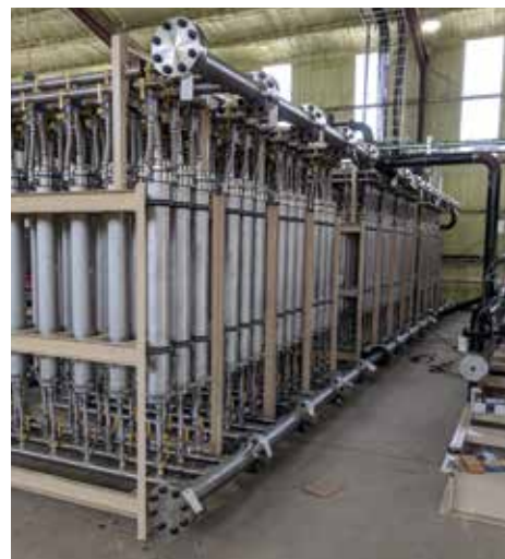
▲ Figure 4. A common membrane separation configuration includes two stages with a recycle stream to maximize methane recovery. The permeate from Stage 1 can be fed to an optional Stage 3 to produce a purified CO_2 stream for reuse.
