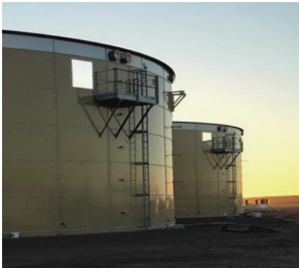
Digesters Under Construction
